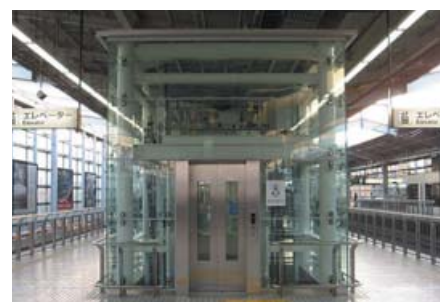
▲ Elevator installation (Kyoto station)
